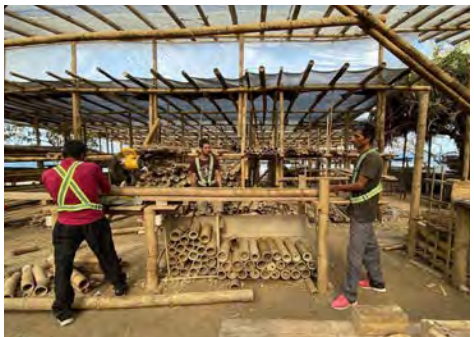
5. STORE AND PREFAB PANELS IN WORKSHOP IN EL ASTILLERO
