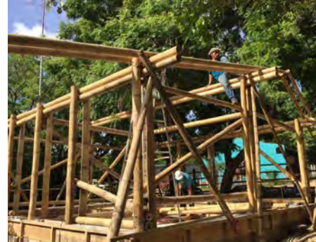
7. ASSEMBLE PANELS IN STRUCTURAL FRAMES
