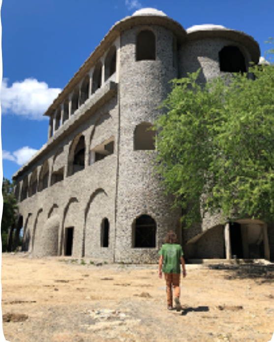
Fig: A new hotel under construction
